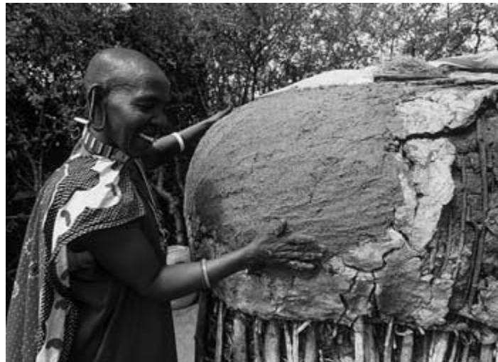
A builder uses a traditional plaster mix incorporating cow dung to maintain her house. Photo: Practical Action / Neil Cooper.
