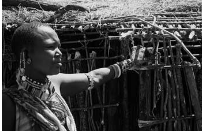
A builder pauses by the structural framework of her traditional house before plastering it. Photo: Practical Action / Lucky Lowe.
