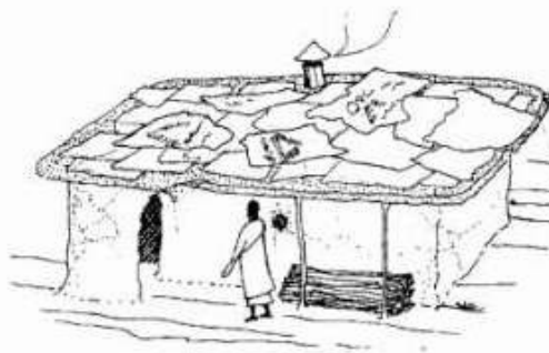
Sprinkling water on the fresh cement to cure it and covering it to keep it damp
