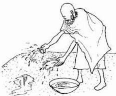
Sprinkling water on the fresh cement to cure it and covering it to keep it damp
