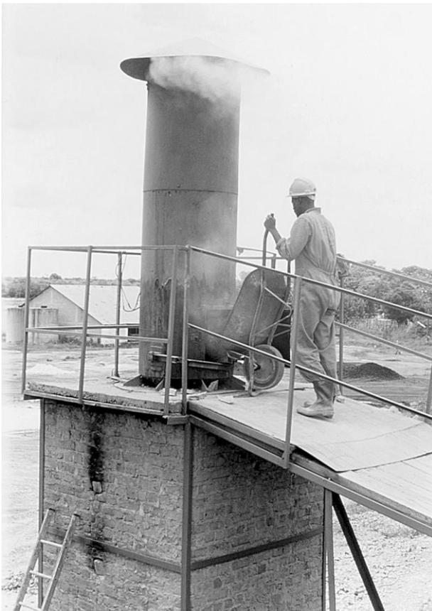
Figure 1: Loading stone/fuel through the hopper at the chimney level, lime kiln, Chegutu, Zimbabwe
