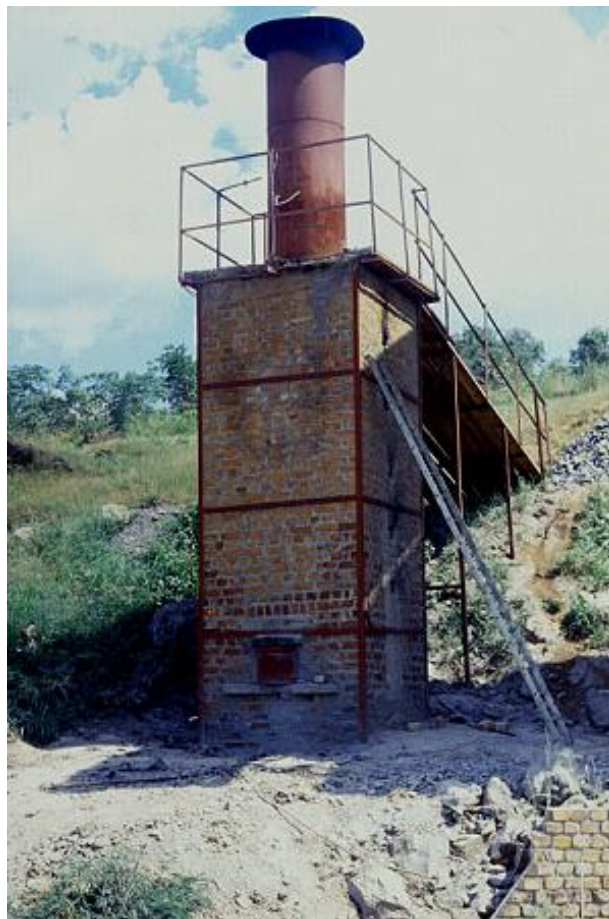
Figure 1: The vertical shaft kiln built for Practical Action in Chegutu, Zimbabwe. Photo: Kelvin Mason/ Practical Action.
