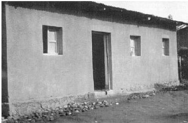
Figure 1: house plastered with lime-pozzolana mix, Rwanda.
