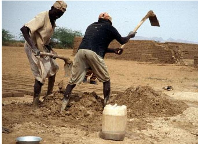
Figure 1: Preparation and mixing of cow-dung bricks.
