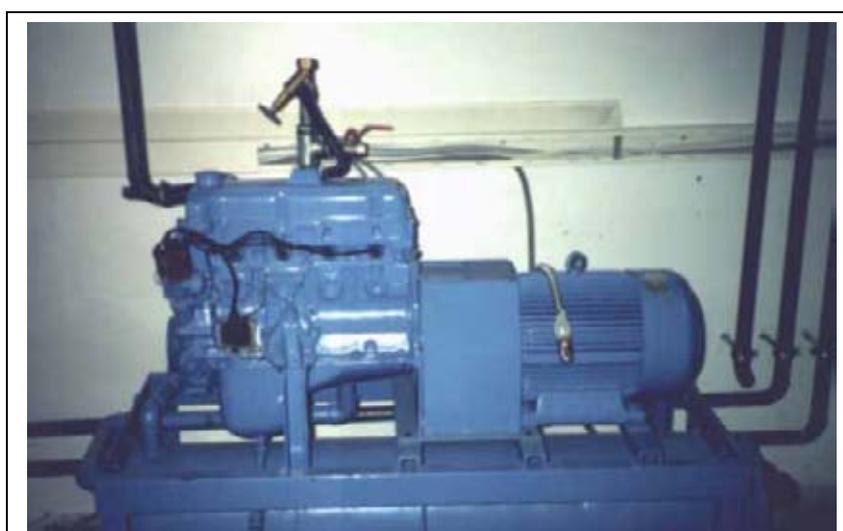
**Figure 47: Co-generation unit (electricity and heat utilisation)**
