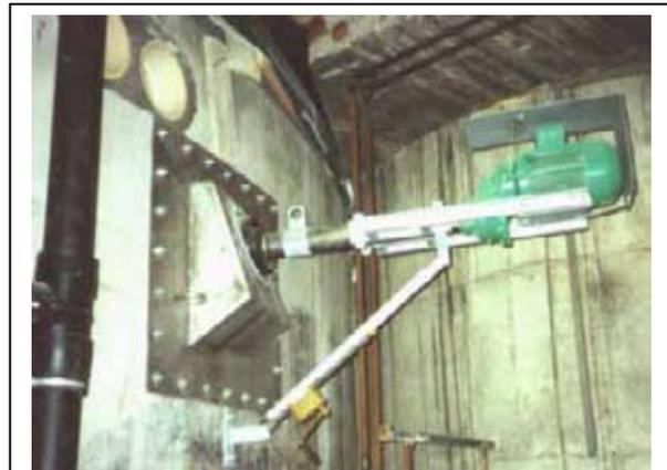
**Figure 19: Stirring device for a european biodigester**
