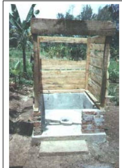
**Figure 16: Toilet (under construction), directly connected to the plant**
