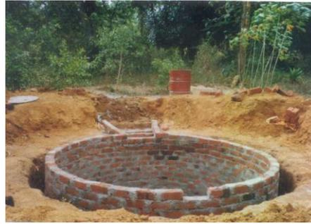
Figure 11: Completed tank before plastering
