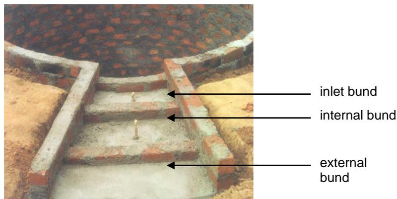
Figure 8: Bunds of the inlet before plastering
