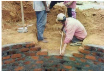
Figure 6: Measurement taken for the inlet construction
