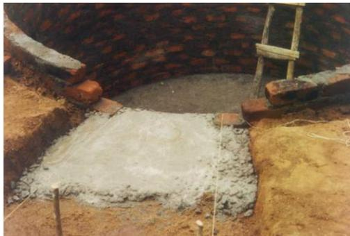
Figure 7: Concrete base for the inlet construction
