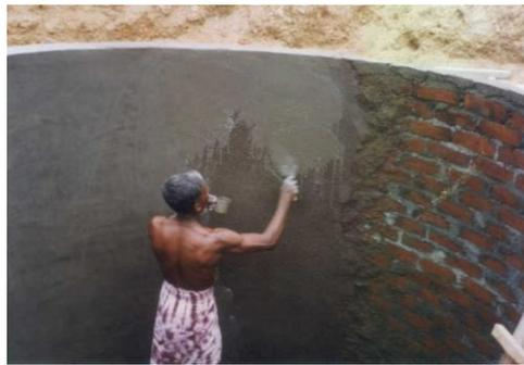
Figure 12: Plastering the tank
