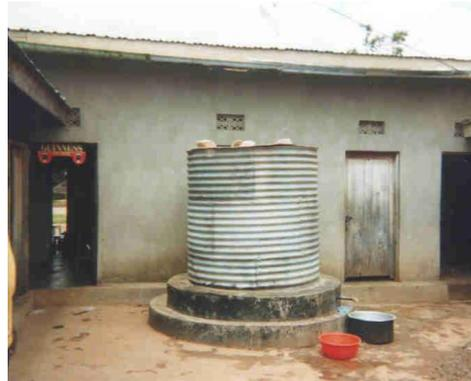
**Figure 4b:** A corrugated iron RWH tank in Uganda
