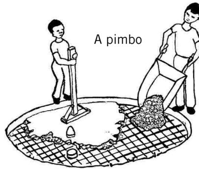
Figure 9: The mesh is covered with more concrete
